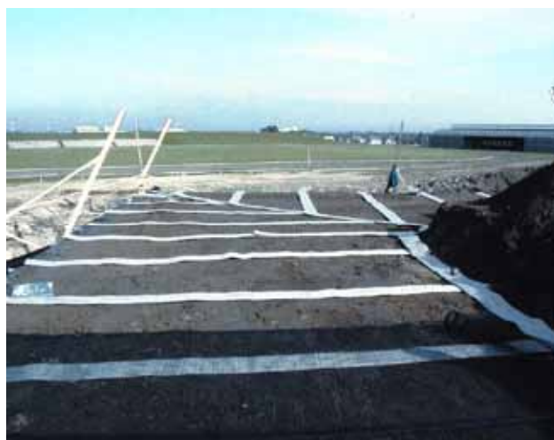
Photograph 1. Installation of horizontal drains
