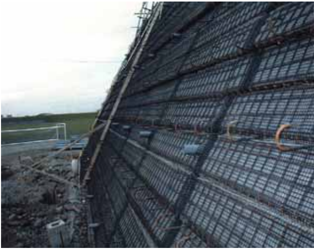
Photograph 2. View of the reinforced banking structure 1
