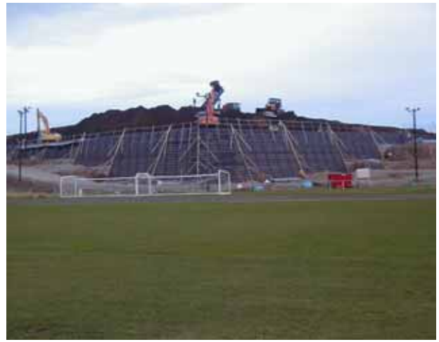
Photograph 3. View of the reinforced banking structure 2
